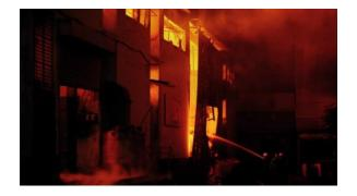
Picture 1: Ali Enterprises Factory. Pakistan's worst industrial accident occurred on September 11, 2012, when a fire tore through a textile factory complex in Karachi. Barred windows and locked exits trapped workers in the four-story building. The fire was caused by short circuits in the equipment. **Damage:** More than 300 workers were killed.
